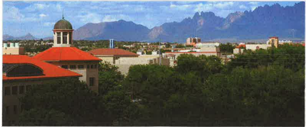
Through Ameresco's partnership with NMSU, energy conservation measures were installed in 46 buildings, saving the University over $1.3 million annually.
